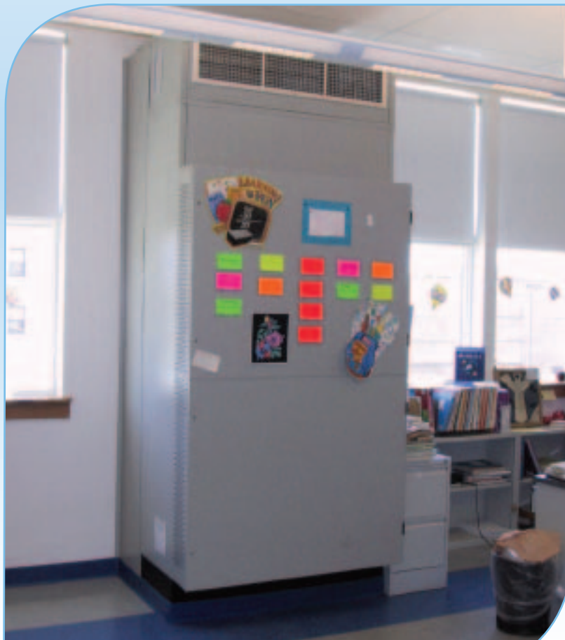
The Marvair Scholar II heat pump, which allowed the school system to keep construction costs under $14 per square foot, also serves as a showcase for student art.
