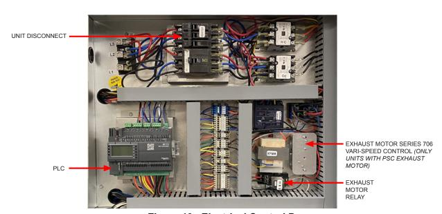
Figure 10. Electrical Control Box
