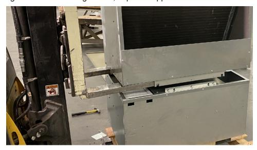
I. After installation of the Scholar unit, install the duct flanges and side panel grommets.
